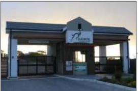
WEST GUARD HOUSE
